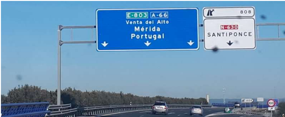
Route 66 to the Extremadura!
